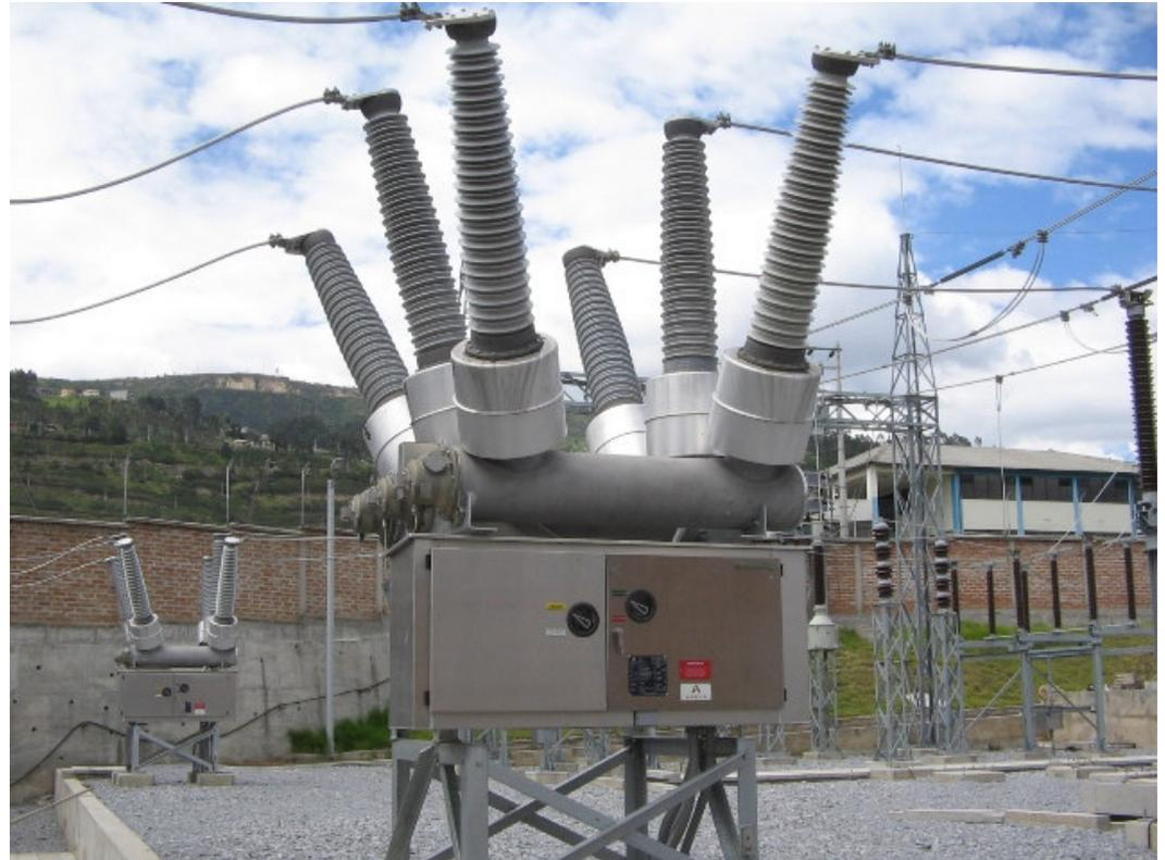
DISYUNTOR EN SF<sub>6</sub> MARCA AREVA , 145 KV, 1250 A
